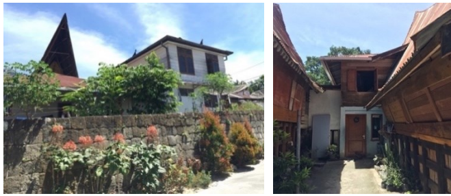
Figure 10. Modern buildings which are built at the back of the traditional one.
